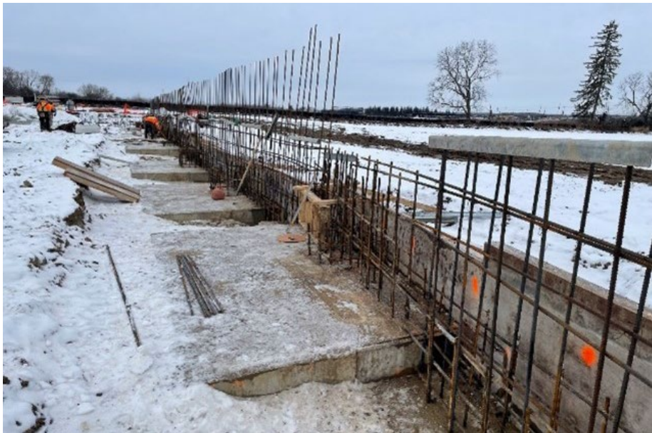
Arena B Wall Reinforcement
