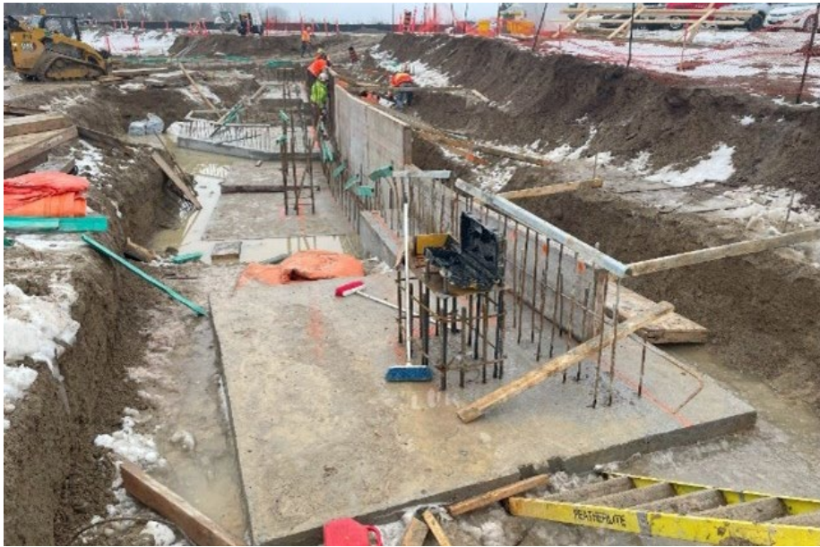
Arena A North Footings
