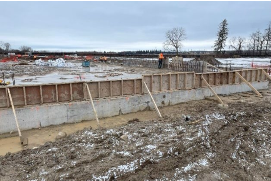
Arena B Wall Formwork
