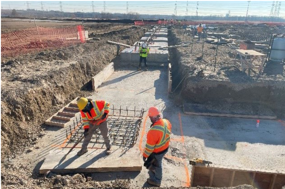
Arena B Footings
