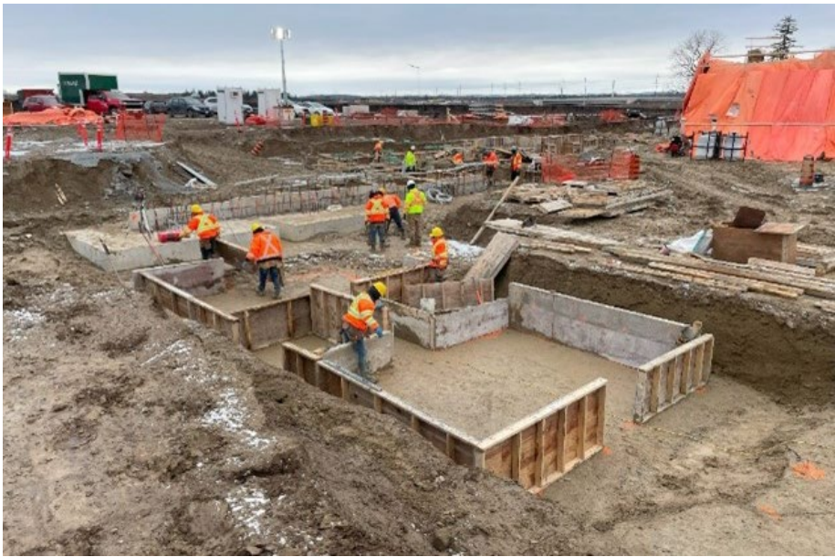
Arena A Northwest Footings
