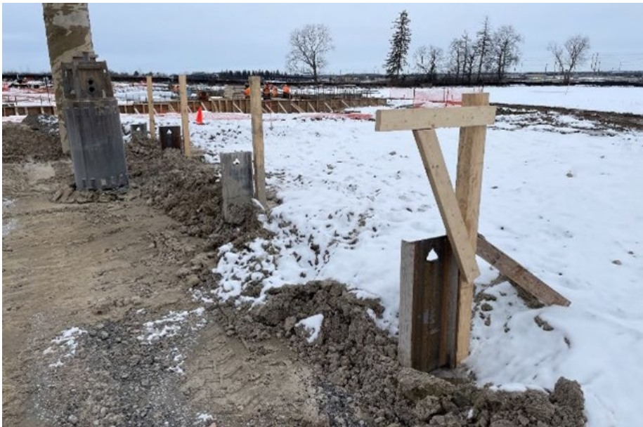
Pool Shoring Installation
