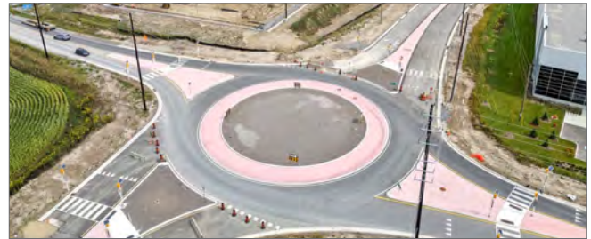
Work continues on the Mid-Arterial Roadway
