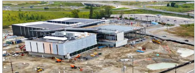
Progress continues on the Whitby Sports Complex
