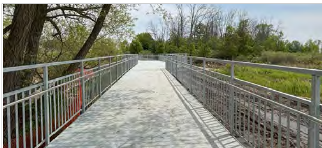
Newly improved Corbett Creek section of the Waterfront Trail
